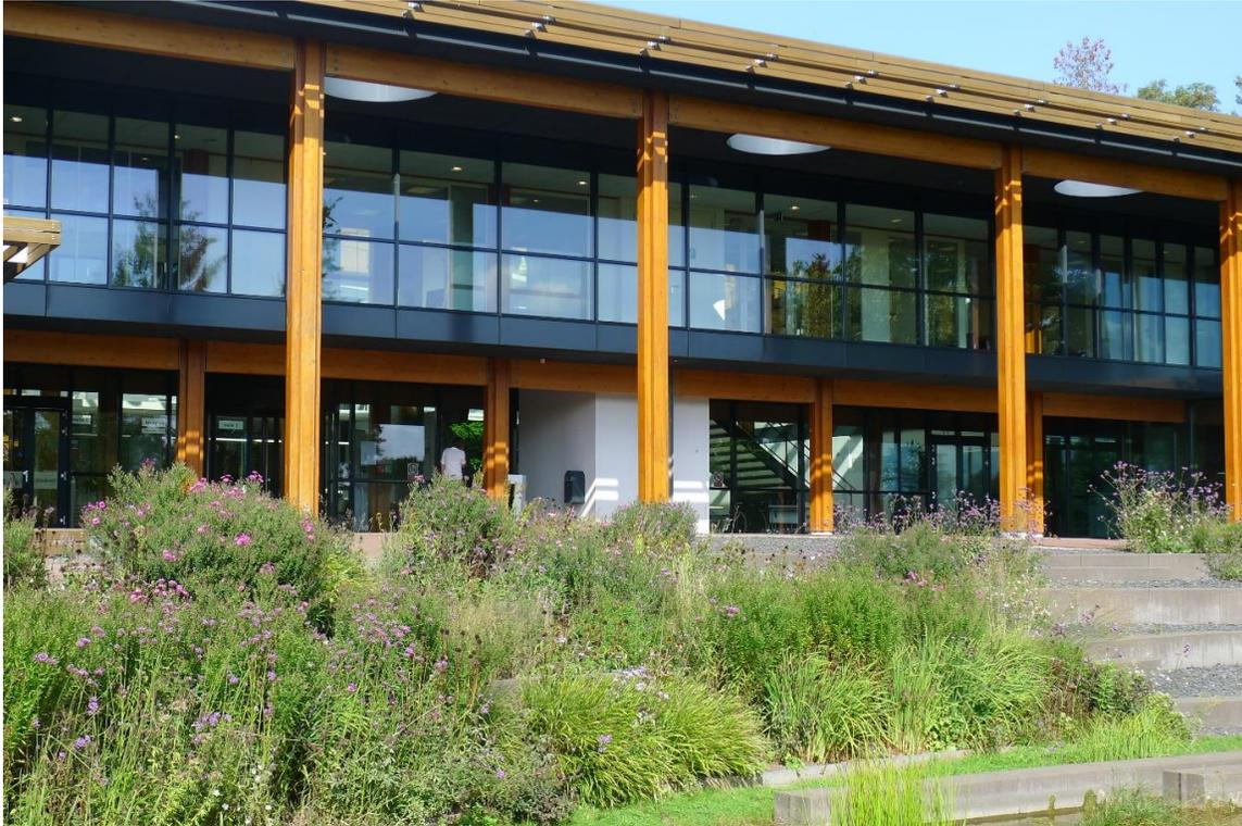
The extension to Brummen Town Hall in the Netherlands incorporates a timber structure, solar gain and is designed for full deconstruction and material reuse. © Clive Bowman, Zero Waste Scotland
